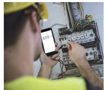
Electric Power Inspection
