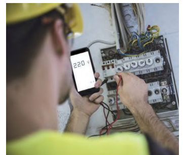
Electric Power Inspection
